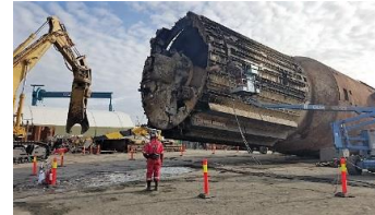
Gullfaks SPM cutting at slipway
